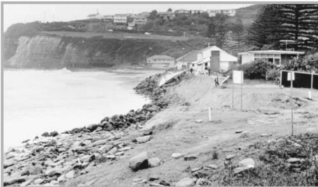
**Fig. 3.19** A) Undermining and collapse of beachfront houses at Bilgola beach, Sydney following the 25 May 1974 storm.
