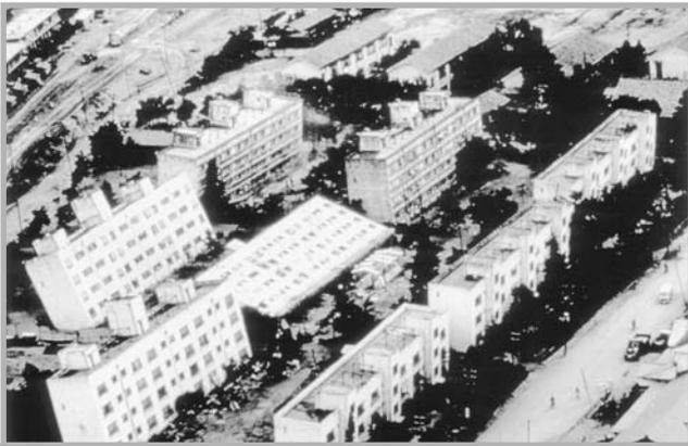
**Fig. 10.10** Liquefaction following the 16 June 1964, Niigata, Japan, earthquake. These workers' apartments suffered little damage from the earthquake, but toppled over because of liquefaction of unevenly distributed sand and silt lenses on the Shinano floodplain. Horizontal accelerations were as low as 0.16 per cent  $g$ . The buildings subsequently were jacked up and re-occupied (photograph courtesy of the United States Geological Survey, Catalogue of Disasters #B64F16-003).
