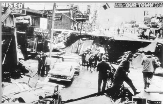
**Fig. 10.5** Head scarp of one of numerous landslides that developed in Anchorage, Alaska, during the 27 March 1964 earthquake. Sand and silt lenses in the Bootlegger Cove Formation liquefied causing loss of soil strength (photograph courtesy of the United States Geological Survey).
