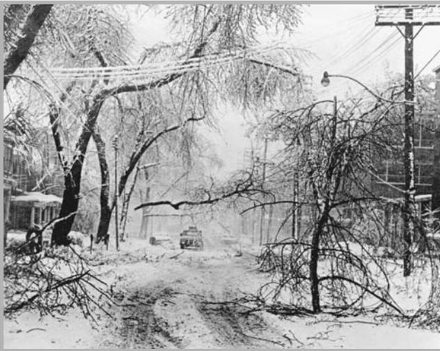
**Fig. 3.24** The effect of freezing precipitation and wet snow on wires and tree branches in Ontario, Canada (photograph from Canadian Atmospheric Environment Service).
