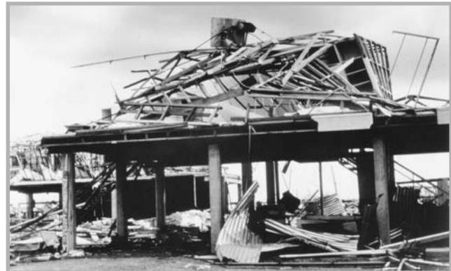
**Fig. 3.9** B) In extreme cases, the high winds progressively peeled off the complete building, leaving only the iron floor beams and support pillars. (Photographs courtesy of Assoc. Prof. Geoff Boughton, TimberED Services Pty Ltd., Glengarry, Western Australia.)
