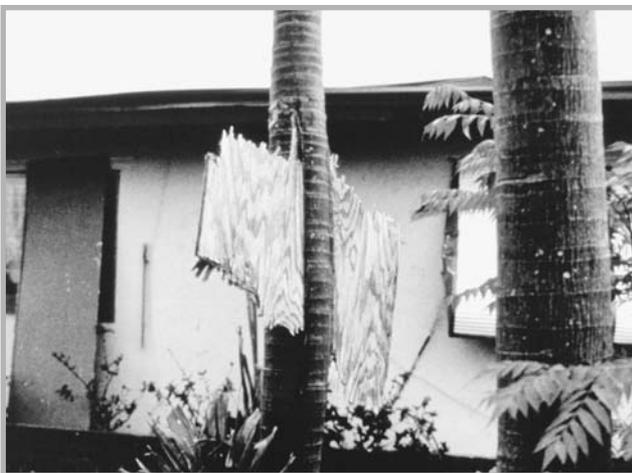
**Fig. 3.8** Sheet of plywood driven through the trunk of a Royal Palm by extreme winds during Hurricane Andrew in South Florida (NOAA, 2003).
