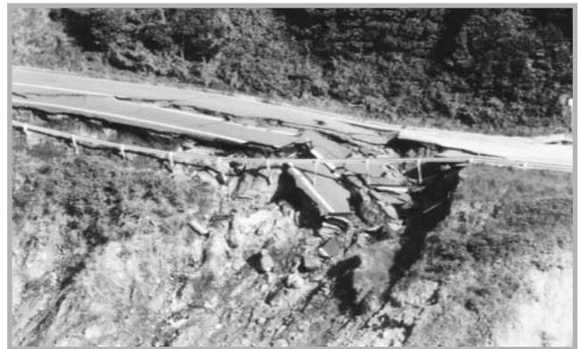
**Fig. 2.9B** B) The same rainfall event in A) caused numerous landslides and washouts that undermined the roadway and adjacent main railway. The total cost in road repairs along this 2 km stretch of coastline was \$A1.5 million. Slippage problems as a result have continued for 15 years (photographs by Bob Webb, courtesy of Mal Bilaniwskyj and Charles Owen, New South Wales Department of Main Roads, Wollongong and Bellambi Offices).
